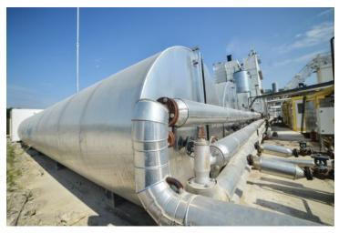
Pipelines transporting mixed asphalt.
